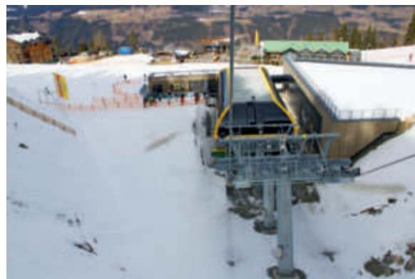
The bottom station of the new Lärchkogelbahn chairlift with 90° loading/unloading was designed with the about same length as the old station so as not to encroach on the ski trail behind it. The 3-rail parking shed on the right is located at ground level next to the bottom station in order to avoid groundwater problems.
