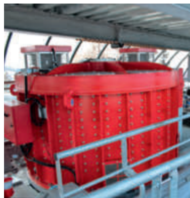
The low-maintenance Leitner DirectDrive in an overhead configuration in the top station
