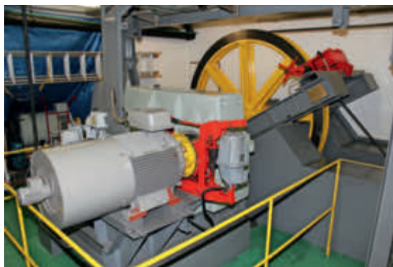
Drive of the Diana funicular installed in 2013 with the asynchronous drive motor and twin-groove bullwheel
