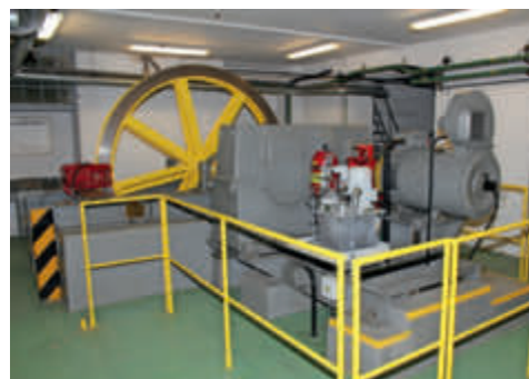
Drive of the Imperial funicular with the twin-groove bullwheel
