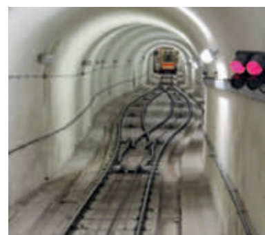
The Abt passing loop on the 127 m long line of the Imperial funicular
